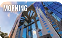
Umeda Sky Building & Osaka Castle
